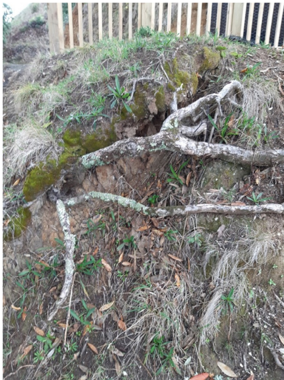
Photograph 6 - 1.2m scarp at top of promontory
