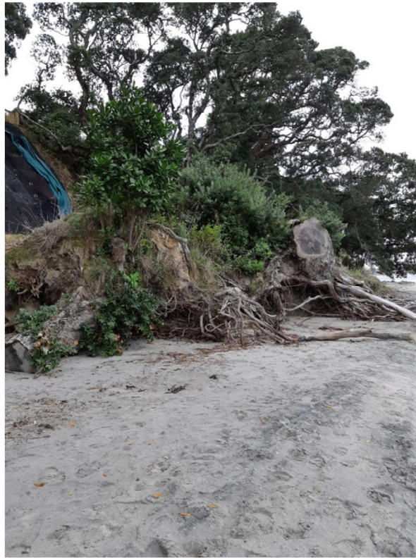
Photograph 13 - Failed Pohutukawa on Foreshore
