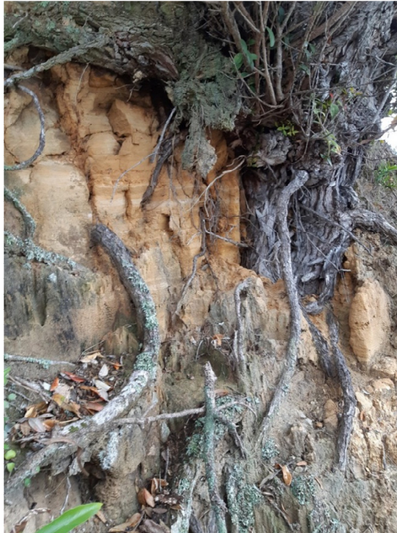
Photograph 5 - Close up view of soils supporting tree
